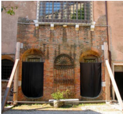
Buttressing & 19th-century brick reinforcement © SGE
